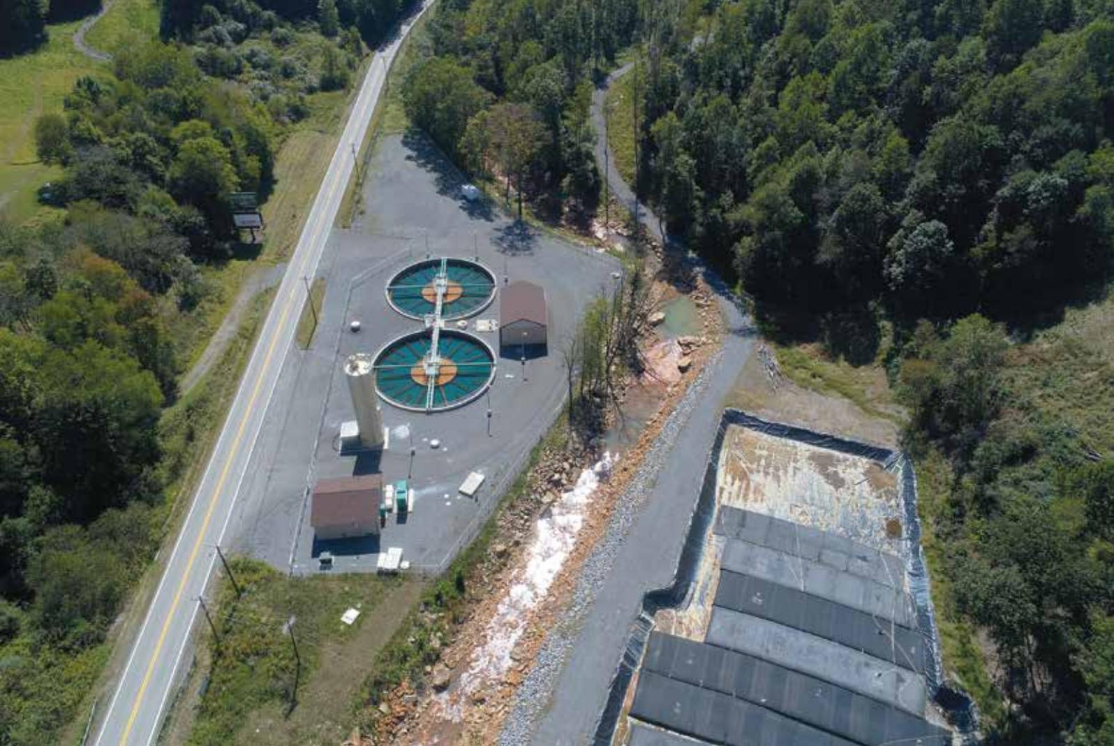
Figure 5. The West Virginia Department of Environmental Protection's Muddy Creek AMD treatment plant near Albright, WV, showing the lime silo and system control building in the lower left, two clarifiers and Geotubes across the creek for collection and dewatering of AMD precipitates.
