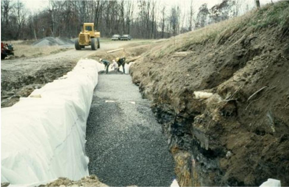
**Figure 5. An anoxic limestone channel being constructed, soon to be covered with plastic sheeting and a soil cover.**
