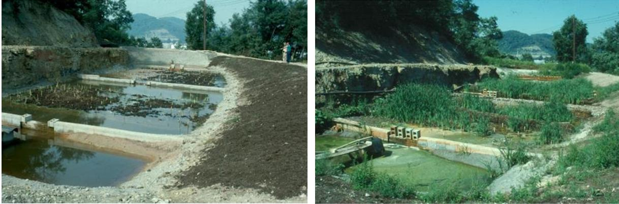
**Figure 3A. A Typha-based wetland immediately after construction in West Virginia. B. the same site, two months later.**
