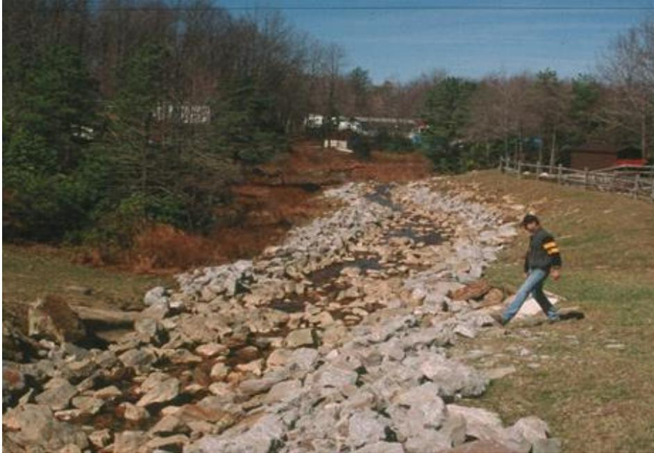
**Figure 4. An open limestone channel (1995)**
