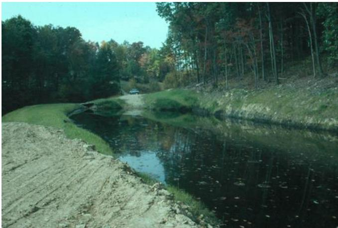
**Figure 6. Construction of an early SAPS in 1995, which has subsequently also been referred to as RAPS, vertical flow ponds, and vertical flow systems. A. Initial placement of the limestone base layer with underdrain piping. B. Compost layer being placed on top of the limestone. C. The system filled with water.**
